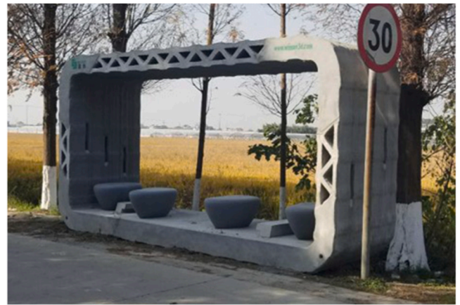
Fig. 9. Extrusion 3DCP printed in 2.5D and turned upright, with post-tensioning different parts for the final shelter. A 3D-printed bus stop shelter made by Chinese company WinSun Construction [89].
