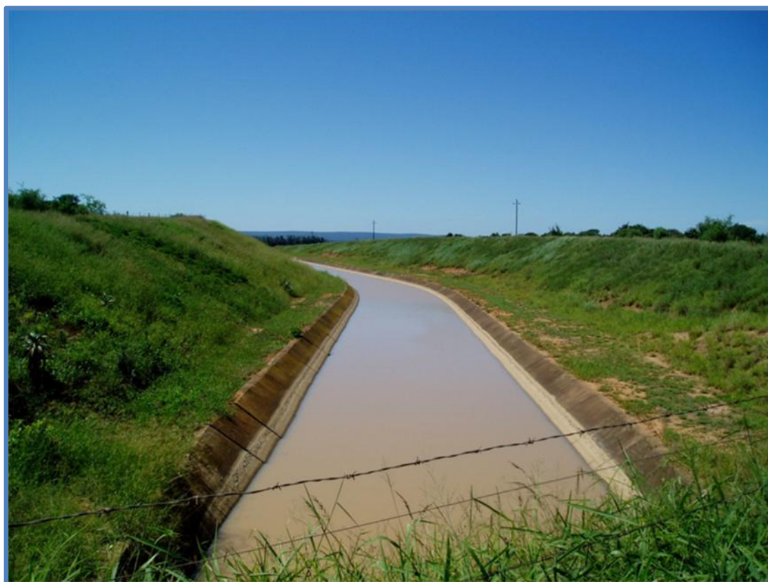
Fig. 10. The Sundays Valley water-transfer canal, which distributes water and fishes from the Orange-Fish-Sundays Inter-Basin Water Transfer Scheme to hundreds of irrigation ponds used for citrus farming. Photo: Darragh Woodford.
