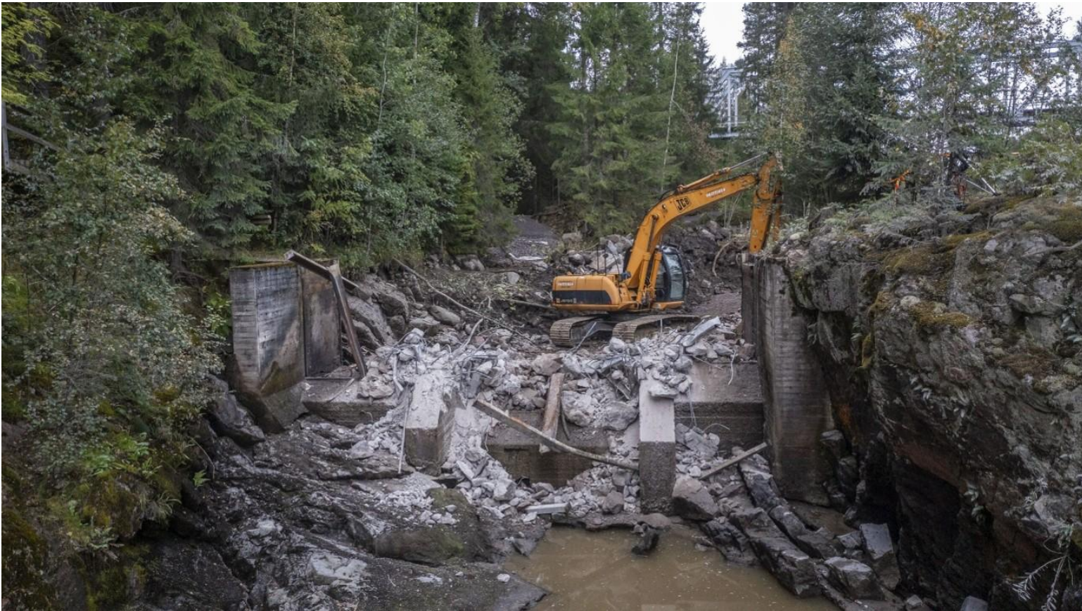
Low-head dam removal from River Hiitolanjoki, Finland, in 2023. Photographed by Mikko Nikkinen – Storymakers
