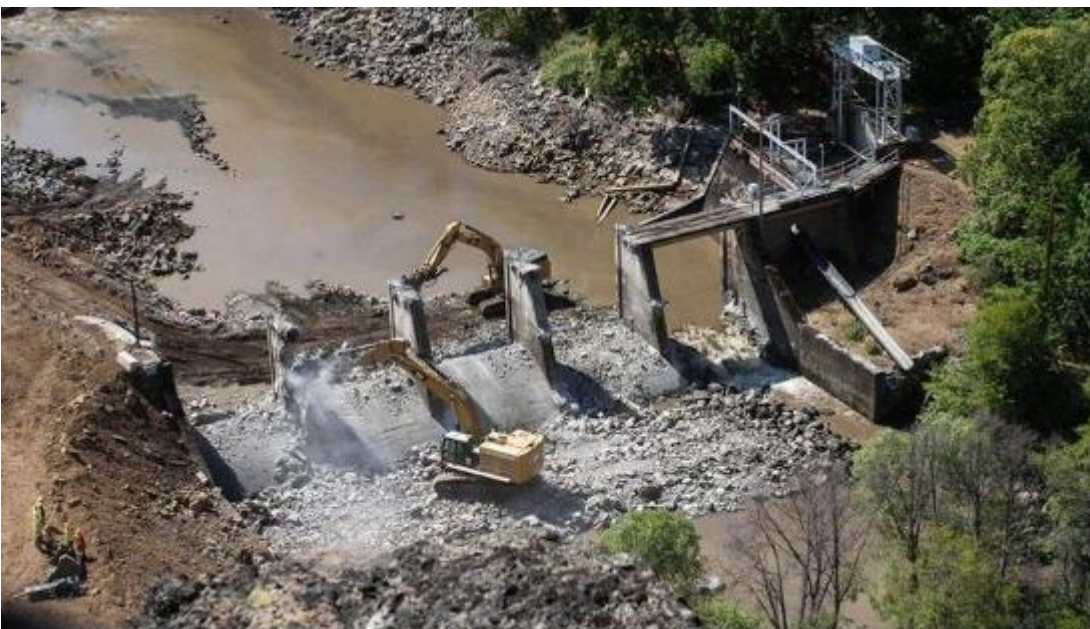
The demolition of the Copco 2 Dam in northern California. Photo credit: Shane Anderson and Swiftwater Films
