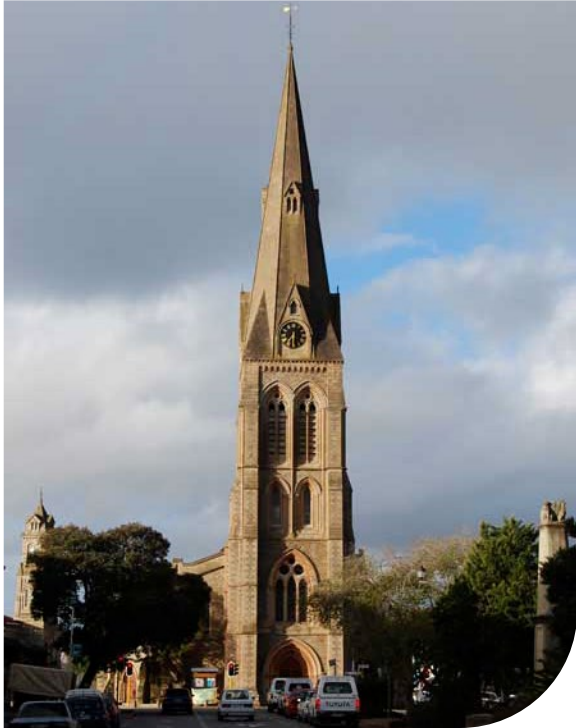
Cathedral Tower (Photograph by William Martinson)
